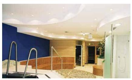
■ Typical ceiling application showing curved bulkheads.
