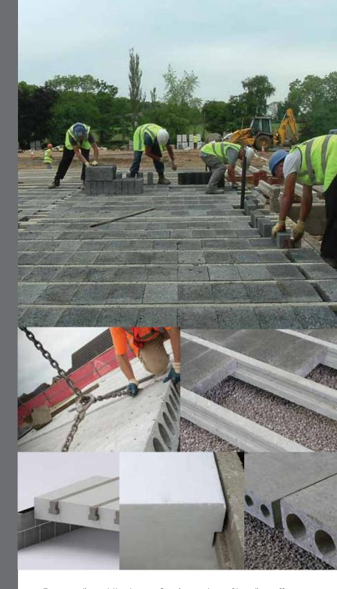
To compliment the beam flooring systems Stressline offer two sections of Hollowcore flooring, with spans in excess of 9 metres, either 150mm deep or 200mm deep to resolve many specification problems. Our hollowcore floors all have a self-weight of 300 kg/m2 which complies to the latest sound regulations.
